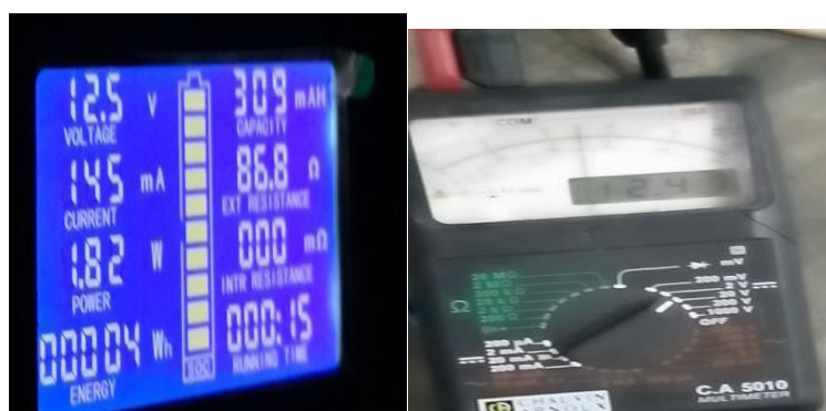
Figure 6. Display of Voltage Values on Measuring Instruments from the Panel Door and Digital Multimeter Measuring Instruments This test involved multiple measurements under varying conditions to ensure data consistency and accuracy. The results were analyzed to identify any system inaccuracies or anomalies. The battery voltage test with the digital multimeter provided insights into
