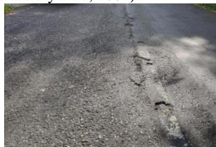
Gambar 8 Pengausan (*Polished Aggregate*) di ruas jalan Weleri – Patean
