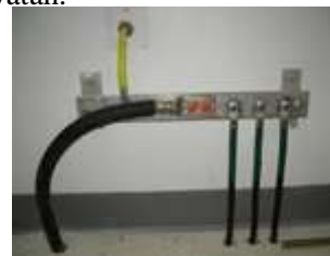
Gambar 16. Grounding System
